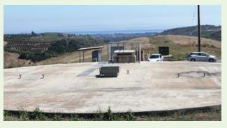
Reservoir aeration treatment was installed at Ellwood Reservoir to treat and remove disinfection byproducts
