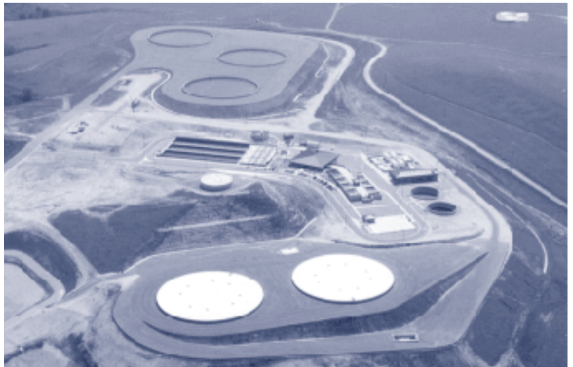
The Polonio Pass facility near Paso Robles treats imported supplies from the State Water Project before delivering the water to Lake Cachuma.
