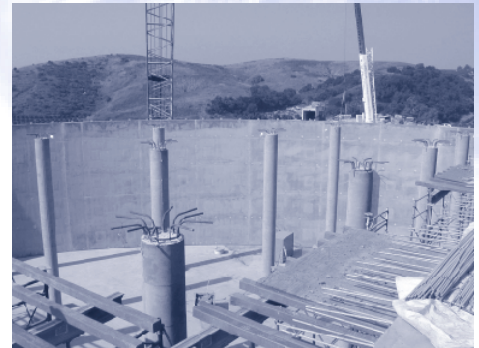
Goleta Water District's Van Horne Reservoir during the construction phase.
